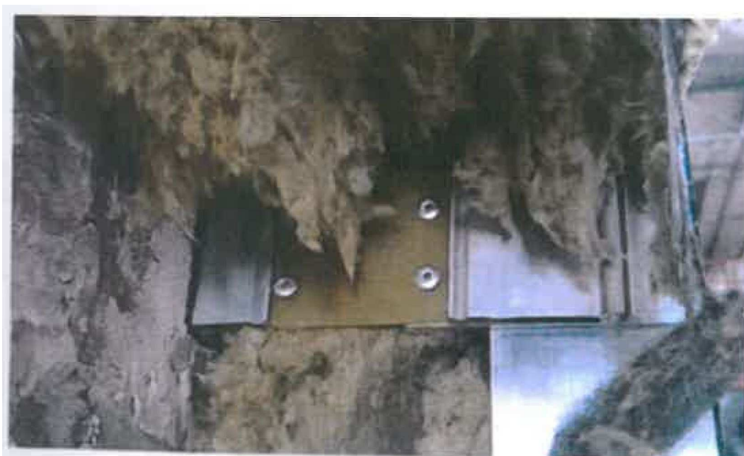
Picture 1 A passive bracket after the test carried out for the purpose of the opinion [3.8] (ITB archive).
